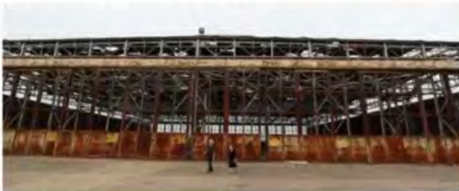
DNAS Maintenance Hangar, 1941
