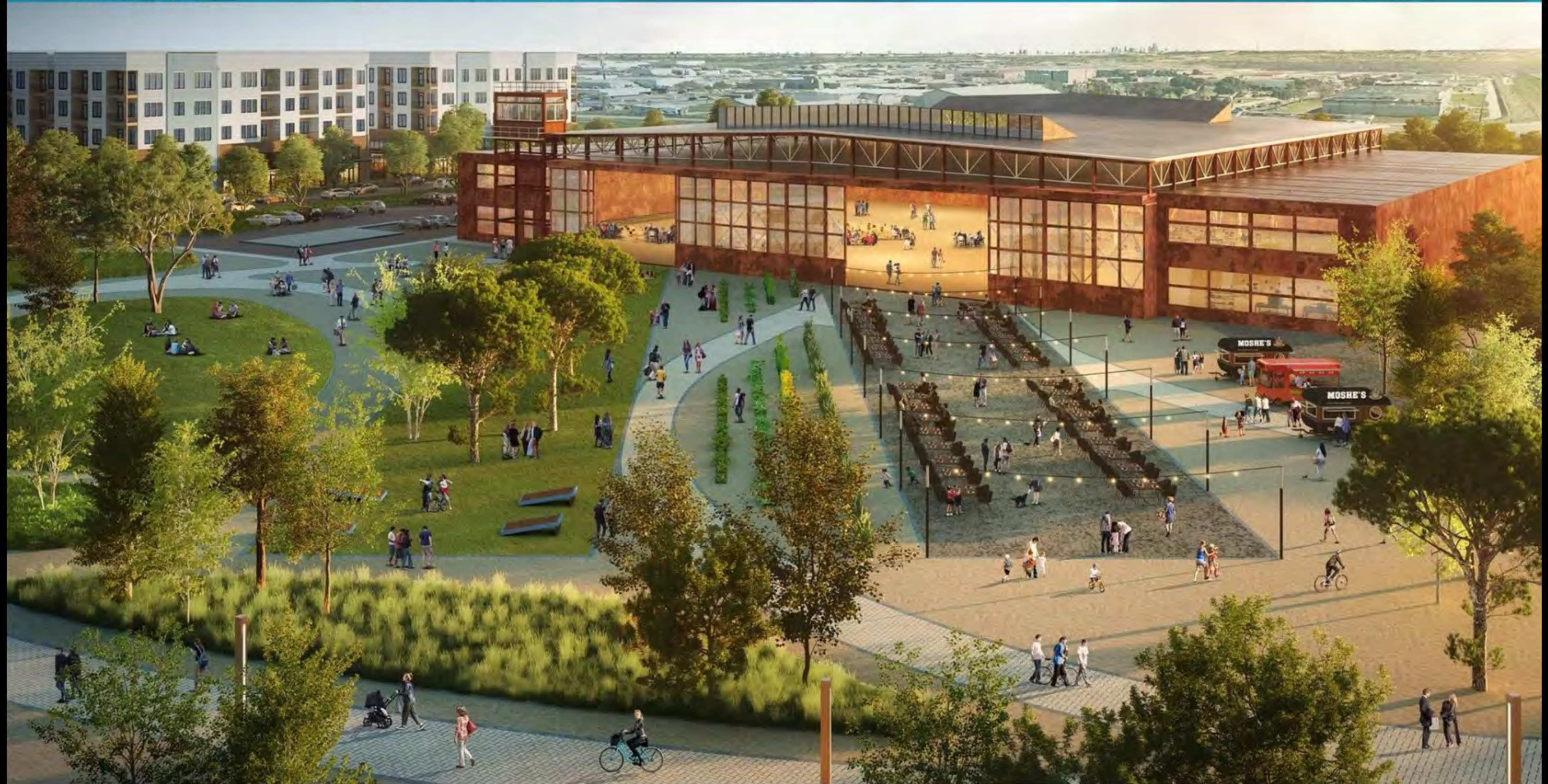
Adaptive Reuse of Dallas Naval Air Station Maintenance Hangar as a Major Cultural Facility or Event Space
