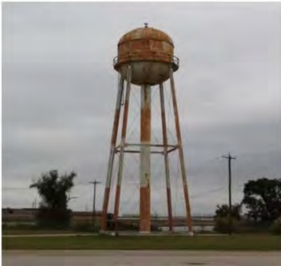
DNAS Water Tower, 1941
