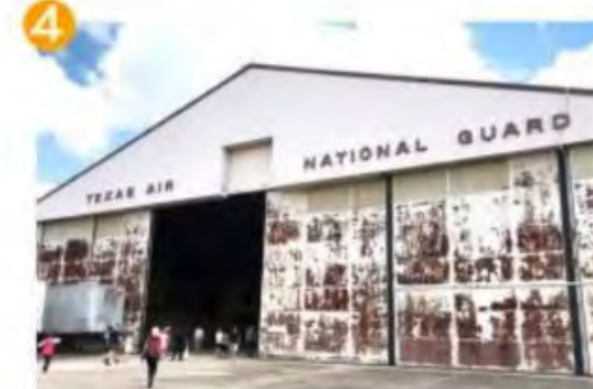
Texas Air National Guard Hangar (1961)
