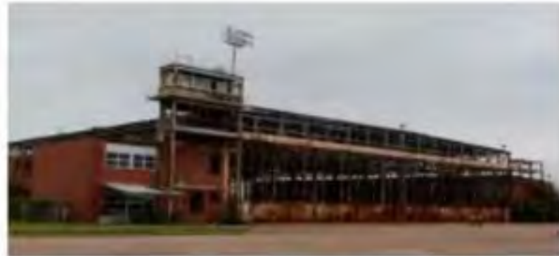
Dallas NAS Maintenance Hangar (1941)
