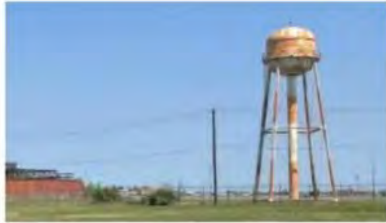
DNAS Water Tower (1941)
