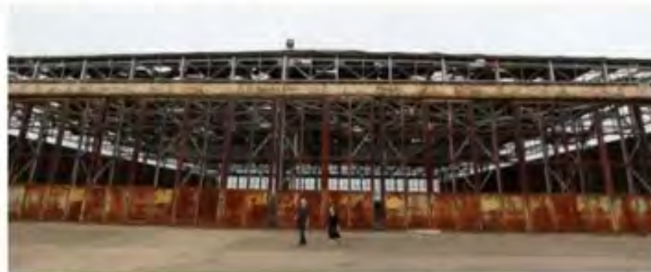
DNAS Maintenance Hangar, 1941
