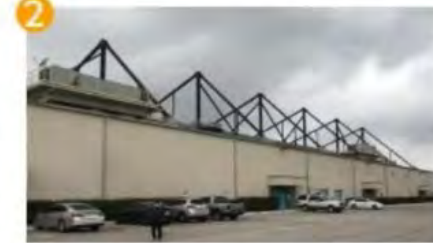
Aircraft Maintenance Hangar (1972-1979)
