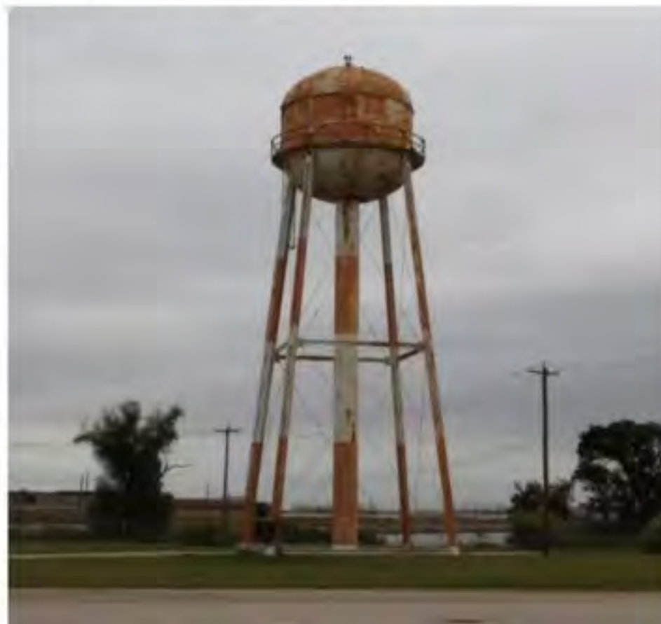
DNAS Water Tower, 1941
