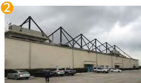
Aircraft Maintenance Hangar (1972-1979)
