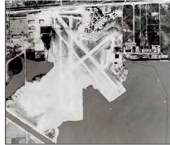
1945 Aerial showing Cottonwood Creek's disconnection to the Lake and the diversion channel being incorporated
