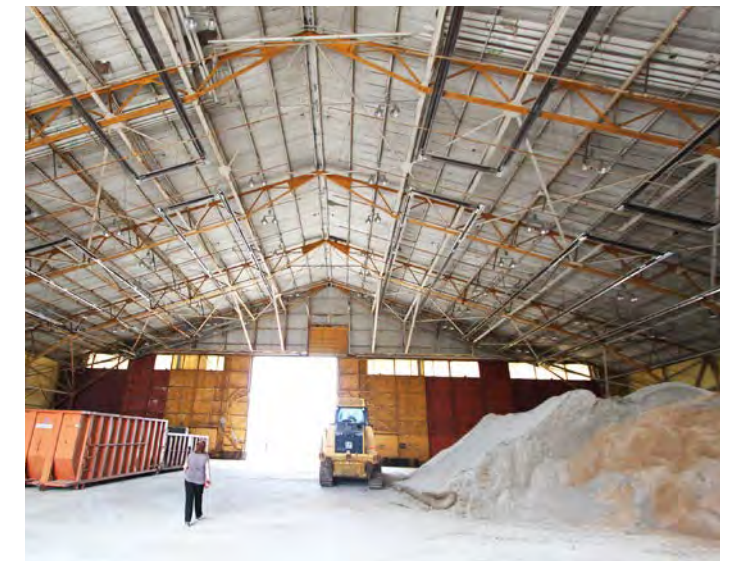
Department of Public Works storage for street repair, 2021
