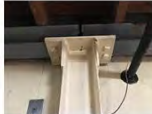
6 Steel Column in Basement
