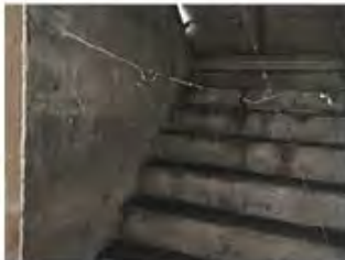
8 Basement Exit Stair
