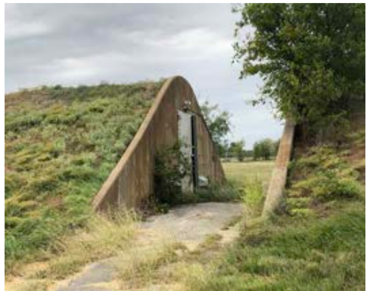
Underground bunker and blast wall
