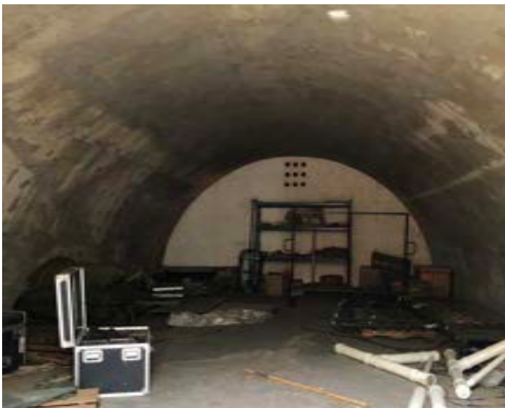
View inside bunker
